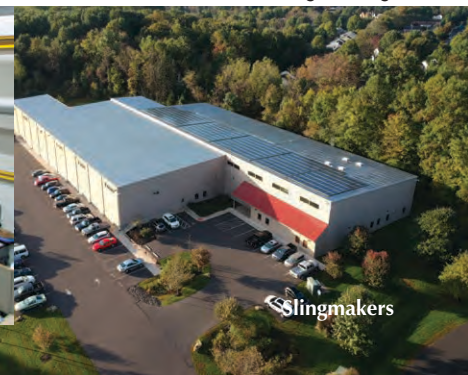
Aerial view of Chant Engineering
