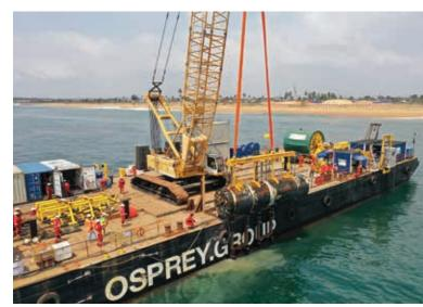
Modulift Custom Subsea Beam Recovering Micro Tunnelling Machine
