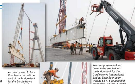
International Bridge. Each floor beam weighs 55,115 pounds and measures 113 feet in length. (Photo Courtesy of WDBA)
