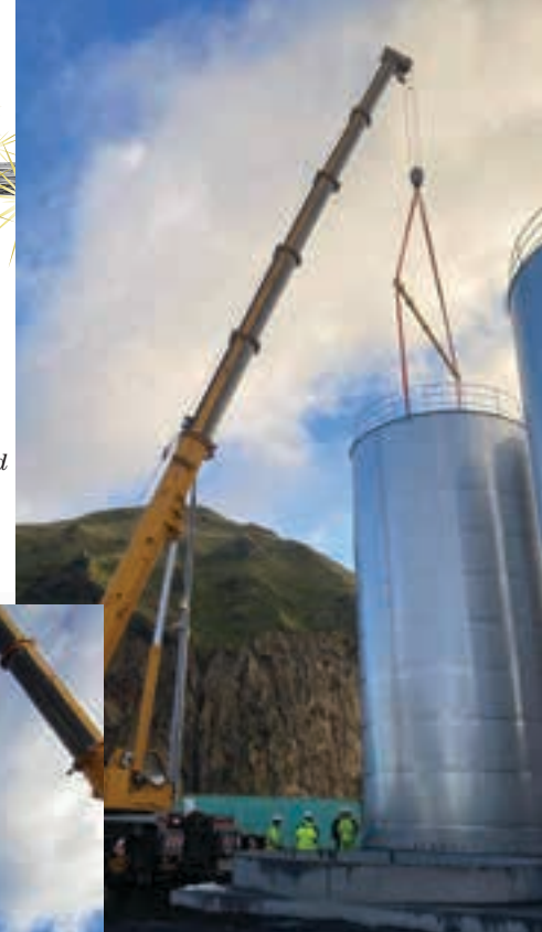
Tank being prepared for lifting
