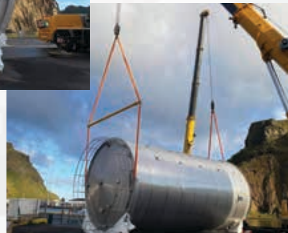
Side view of tank being prepared for lifting
