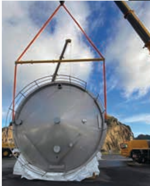
Tank being prepared for lifting
