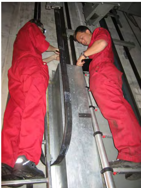
Picture 1: Inspection of an elevator
