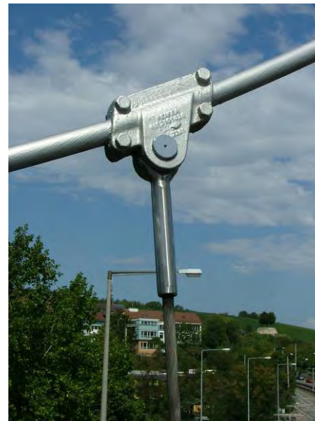
Picture 3: Swaged Terminal on a bridge
