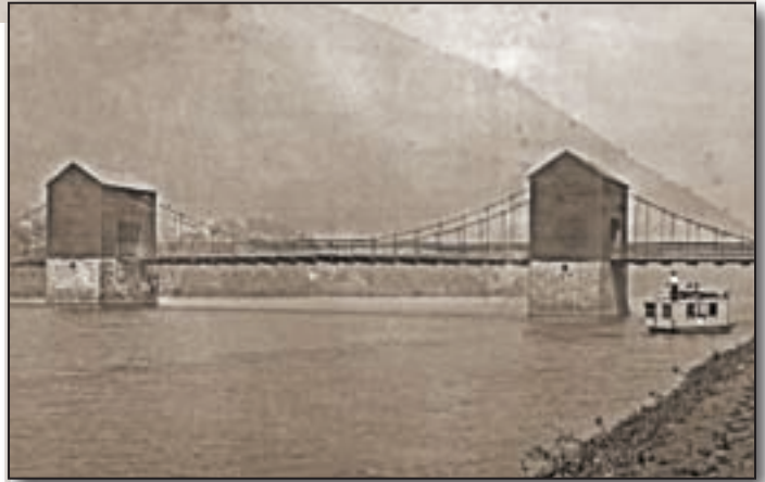
Figure 1 – Lehigh Water Gap Chain Bridge. Central span 160 feet with two half spans 80 feet each. Opened for travel 1826. Dismantled 1933. This photograph was made c. 1900. It is from the collection of the National Canal Museum, Easton PA.
